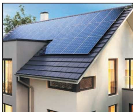
The solar panels are facing south on the roof.
